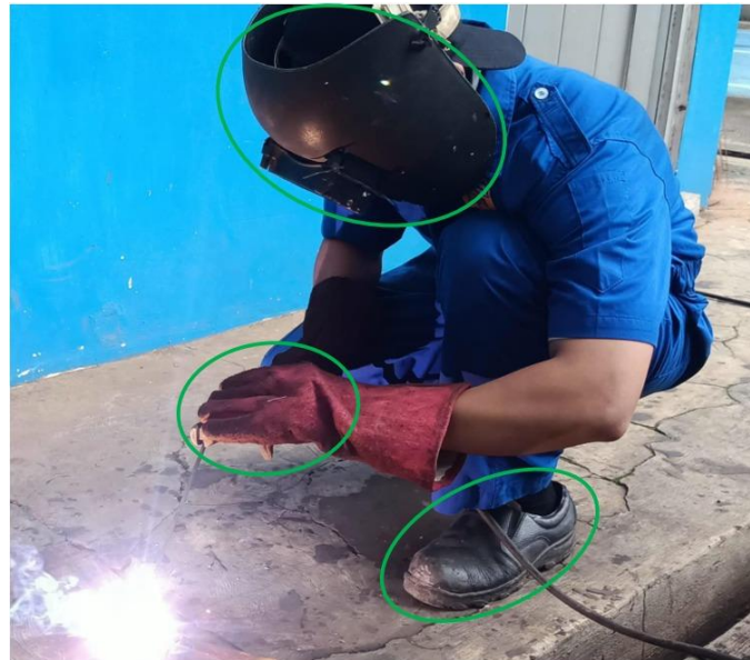
Figure 1. Work Process with SMAW Welding.
