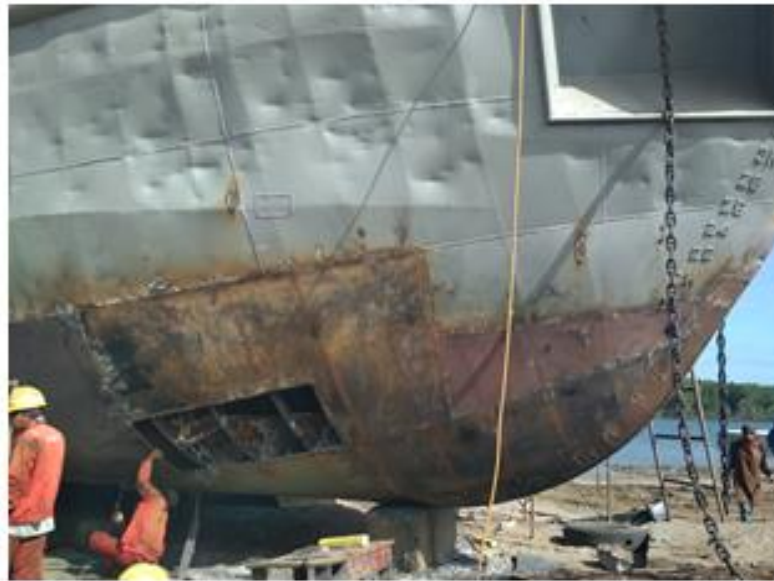
Figure 1. Replating place of the bottom near forepeak
